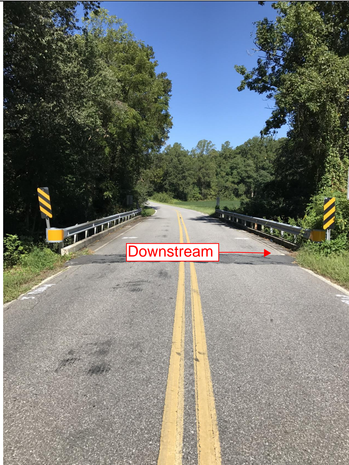
Facing Upstation from End Bent 1 (-L-)
